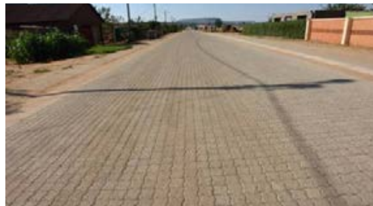
Figure 10.3: Example Paved village roads for improved accessibility using labour intensive pavers. This method promotes the creation of local jobs and transfer of skills to SMMEs within the municipality. This method can be considered for the rural areas.
